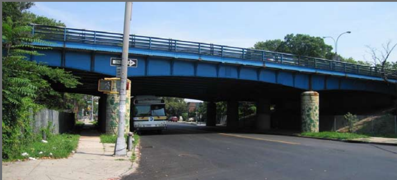
Existing Nostrand Avenue Bridge
