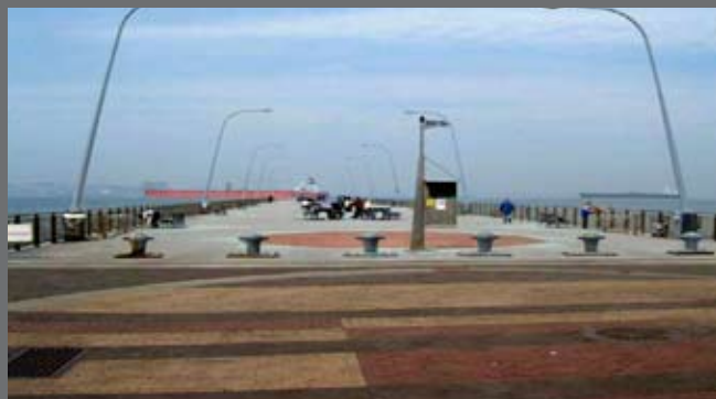
Bay Ridge Avenue Pier
