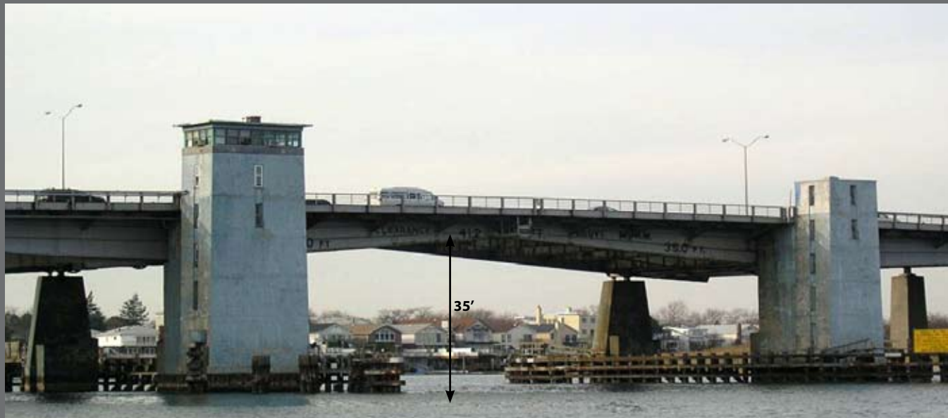
Existing Mill Basin Bridge
