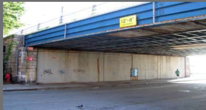
Existing condition of Bay Ridge Avenue Bridge
