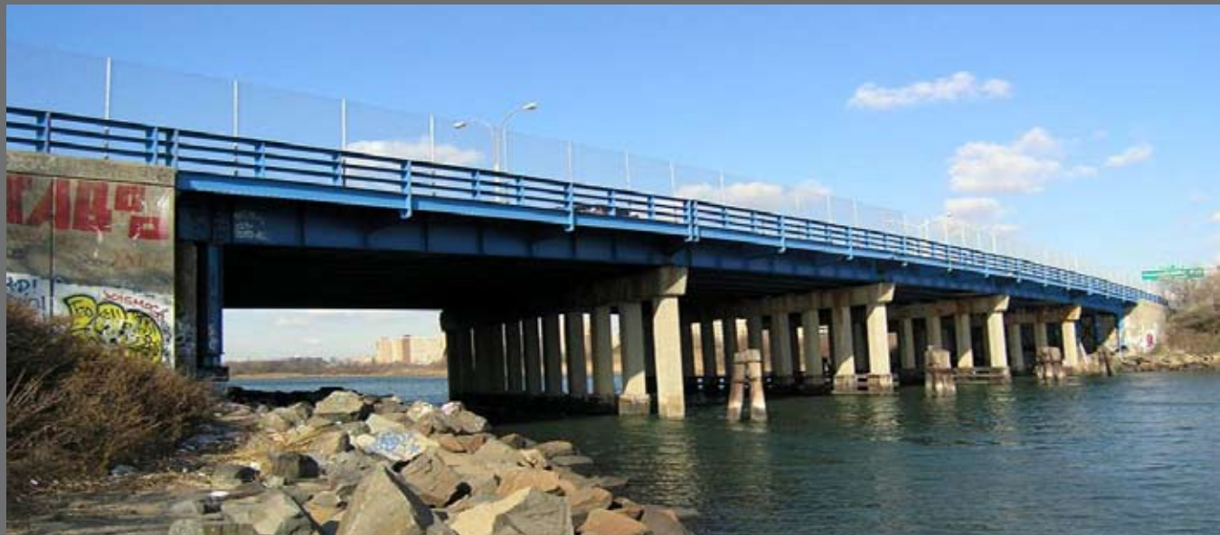
Existing Fresh Creek Basin Bridge
