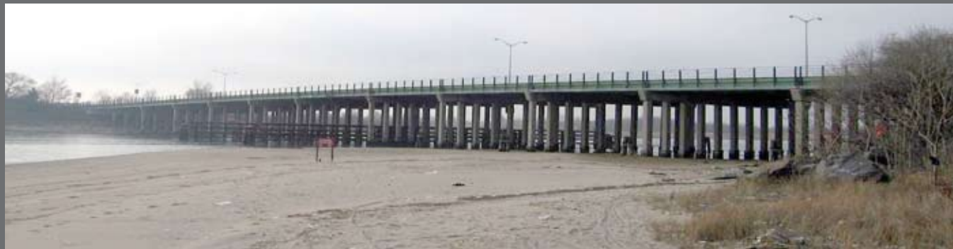
Existing Paerdegat Basin Bridge
