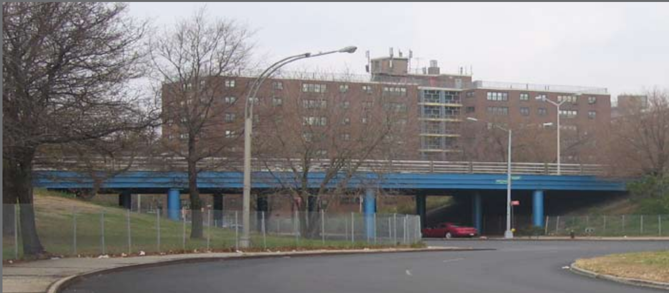
Existing Rockaway Parkway Bridge
