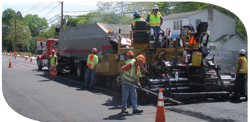
Paving Crew in Action
